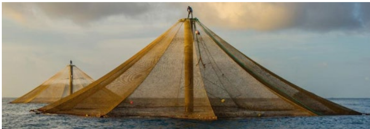
Figure 7 | Two of Open Blue’s InnovaSea SeaStation cages off the Panama coast. The cages are in their fully raised position to allow for net maintenance. Source: Open Blue.
